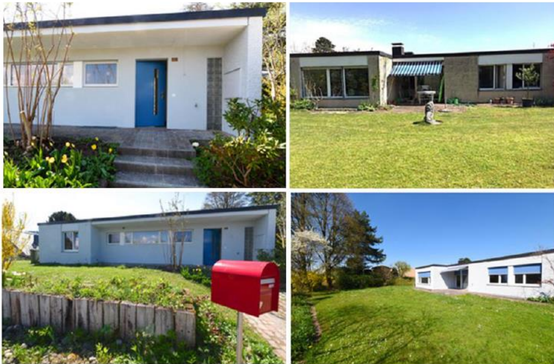
Figure 1: The case study building located in Switzerland, Zurich [9,10].
