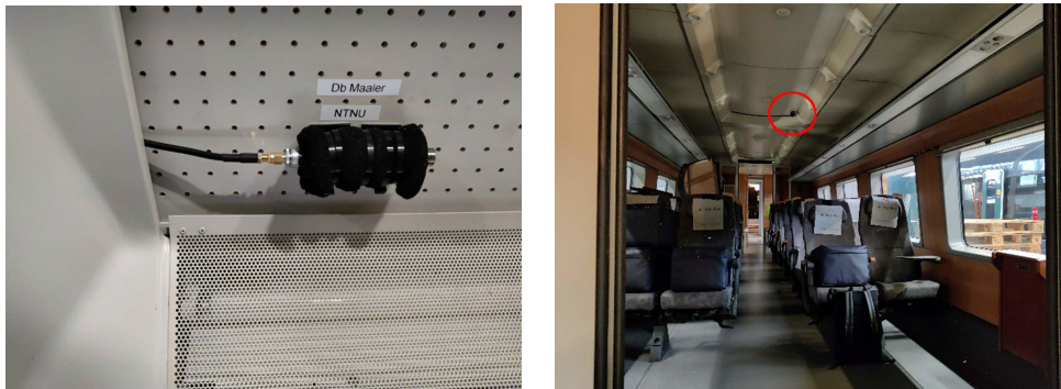
Figure 7: Cabin microphone installation: (a) close-up and (b) location in the passenger cabin.
