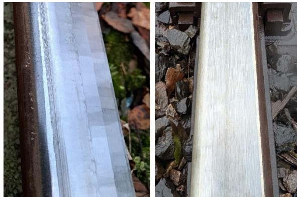
Figure 10: Left - rail surface condition directly after milling (milling grooves visible) with no post processing. Right - rail surface condition after one ATMO pass.
