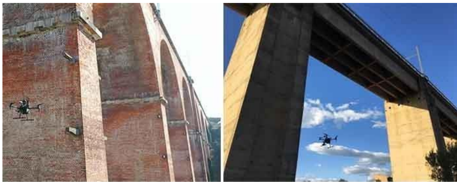
Figure 5: Field activities, inspection of various types of bridges using UAS (drones)
