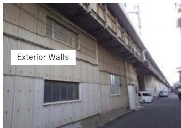
Figure 6: Viaduct with Buildings Located Beneath the Viaduct
