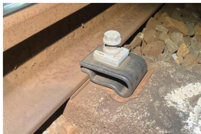
Figure 8: Condition of the rail fastening system several months after trial installation.
