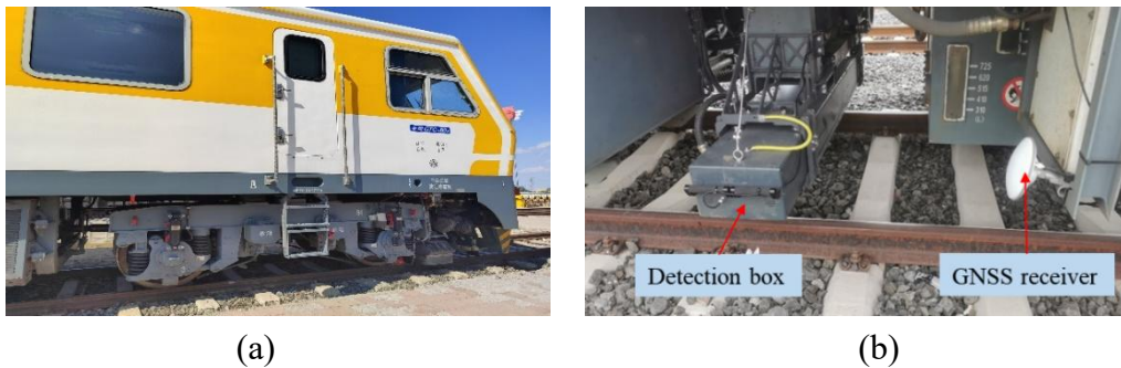
Figure 8: System dynamic installation test. (a) Test vehicle platform; (b) On site diagram.
