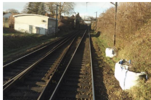
Figure 1.b: Ballast big bags left along train tracks
