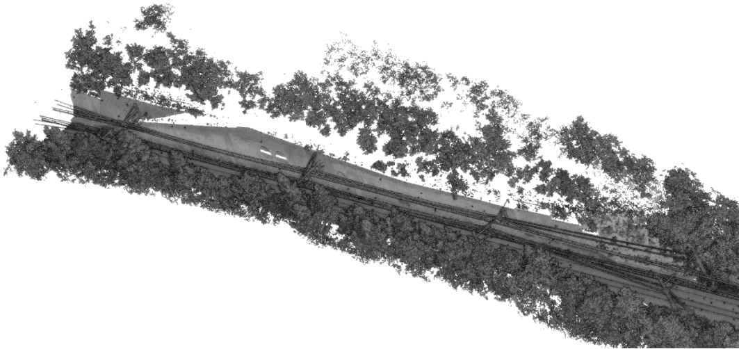
Figure 4. Example of trainborne LiDAR point cloud containing a retaining wall.
