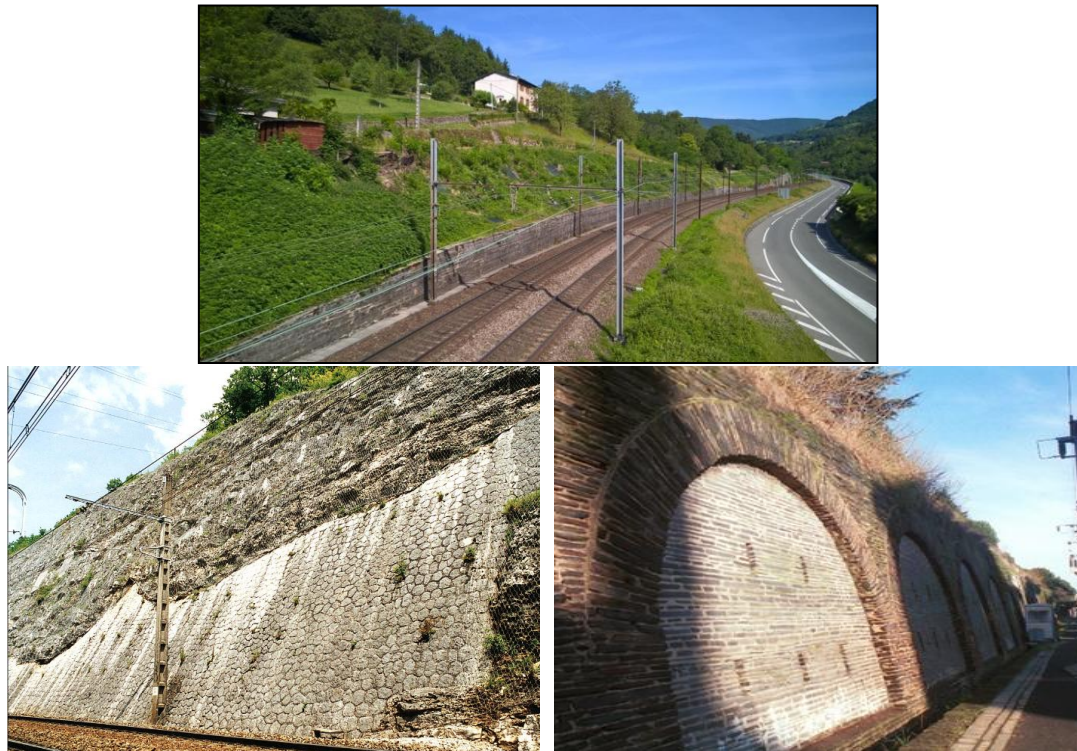
Figure 1. Examples of retaining walls.
