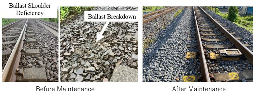
Figure 5: Status before and after maintenance work (ballast spreading)
