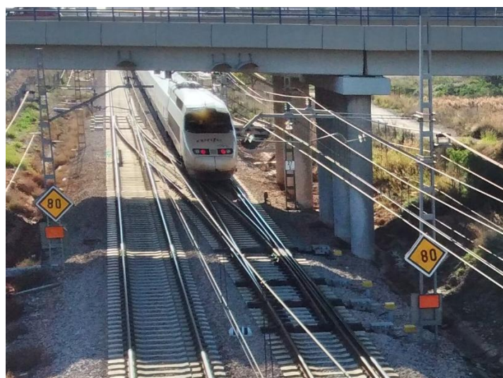
Figure 1: Dual gauge S&C.
