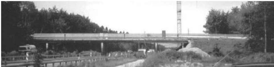
Figure 1: Archive picture of the Z24 bridge [7].
